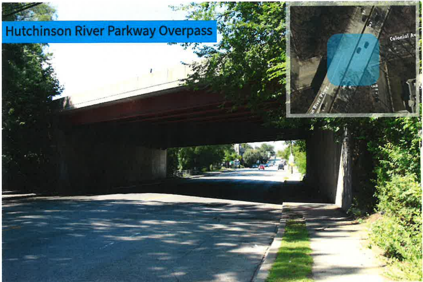
Figure 8: The Hutchinson River Parkway Underpass.
